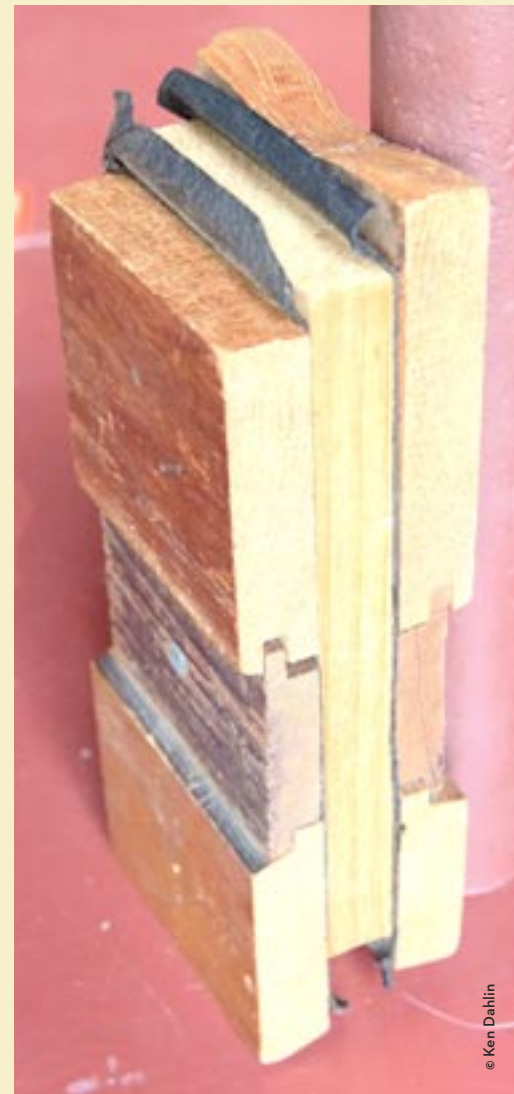
The board-and-batten walls at Jacobs I, Madison, consist of 3 layers of pine wood and 2 layers of building paper.
