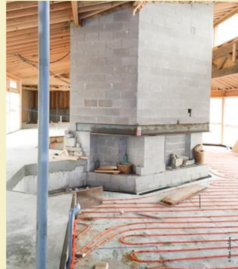
Polybutylene tubing improves the efficiency and reliability of radiant heating.
