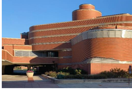
SC Johnson & Son Administration Building
